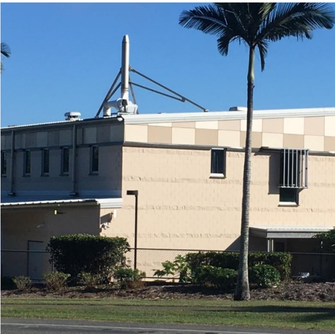
Figure B2: Upgraded roof vent supports
