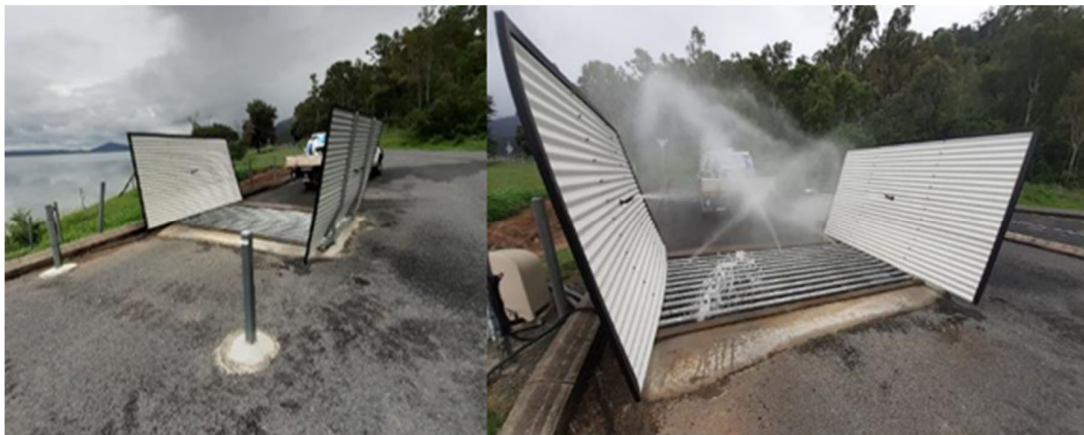
Figure 3: Peter Faust Dam (Proserpine) Automated Washdown Facility
