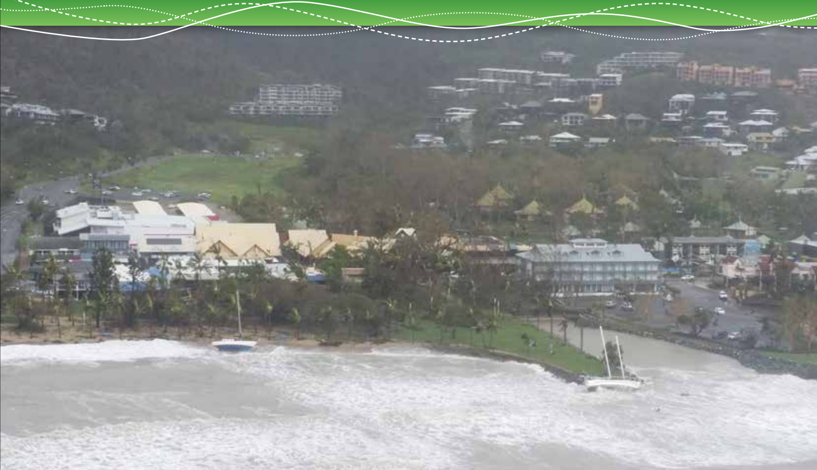
Figure 2: Damage cause by coastal storms, Airlie Beach
