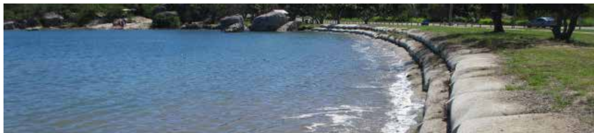
Figure 15: Grays Bay sand bag wall
