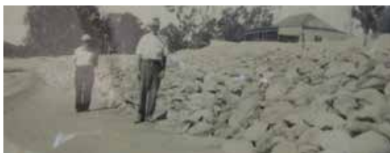
Figure 34b: Queens Beach sea wall from the 1940’s
