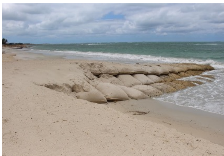
Figure 17: Geotextile groyne on Drummond Cove foreshore (City of Greater Geraldton 2019)
