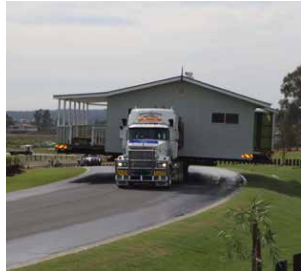
Figure 24: House relocation during Grantham land swap program
