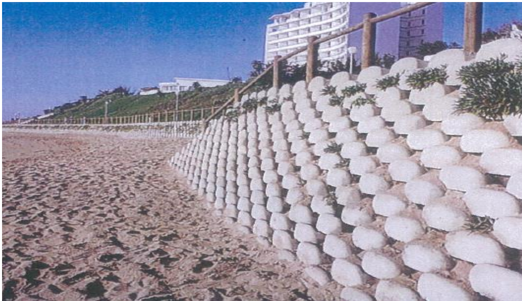
Figure 19: Typical concrete block wall
