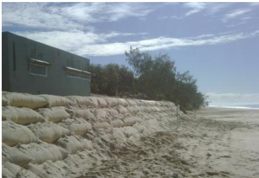
Figure 18: Typical Geotextile Sand Filled Container Wall
