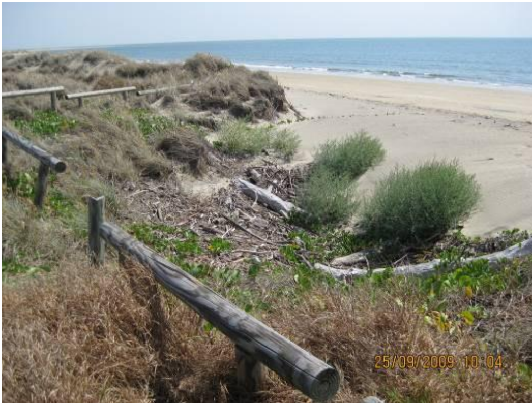
Figure 5. Stormwater discharge point for the Beach avenue drain.
