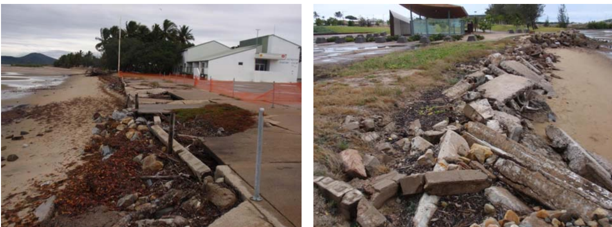
Figure 3.8 : Rubble seawalls either side of the concrete ramp
