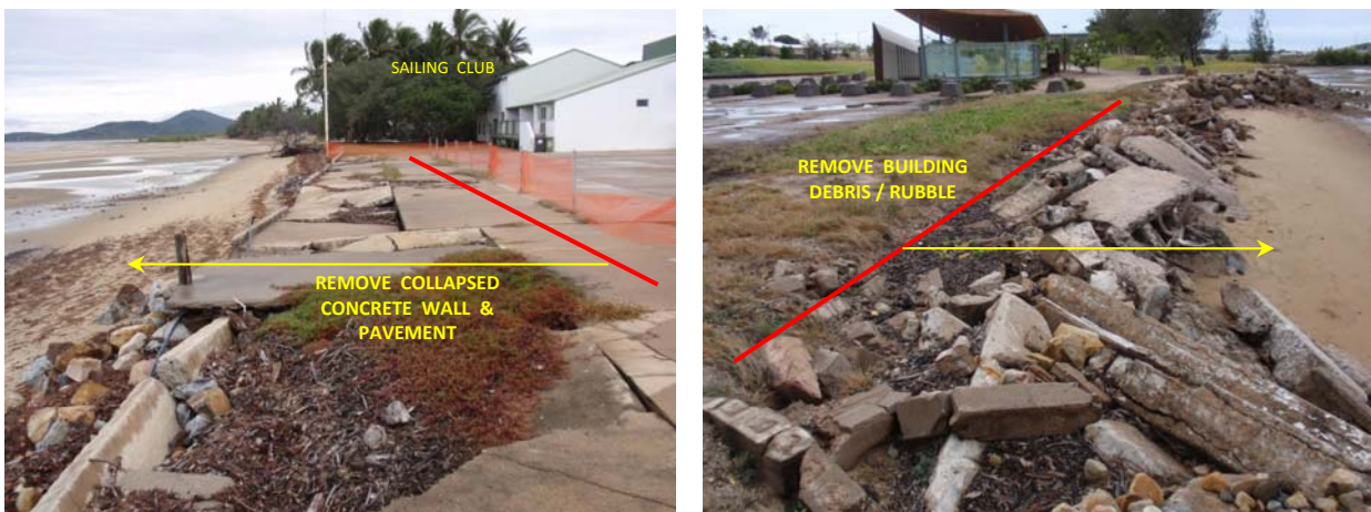
Figure 6.4 : Preparation Works Prior to Beach Nourishment Alongside Concrete Ramp
