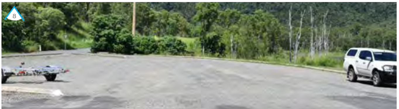
Main Carpark - Insufficient use of line marking and organisation leads to congestion on busy days
