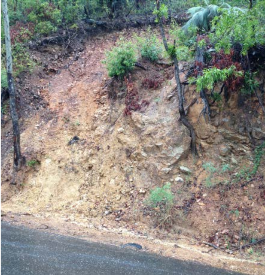
Figure 5-4 Translational landslide removing weaker soils over stronger bedrock
