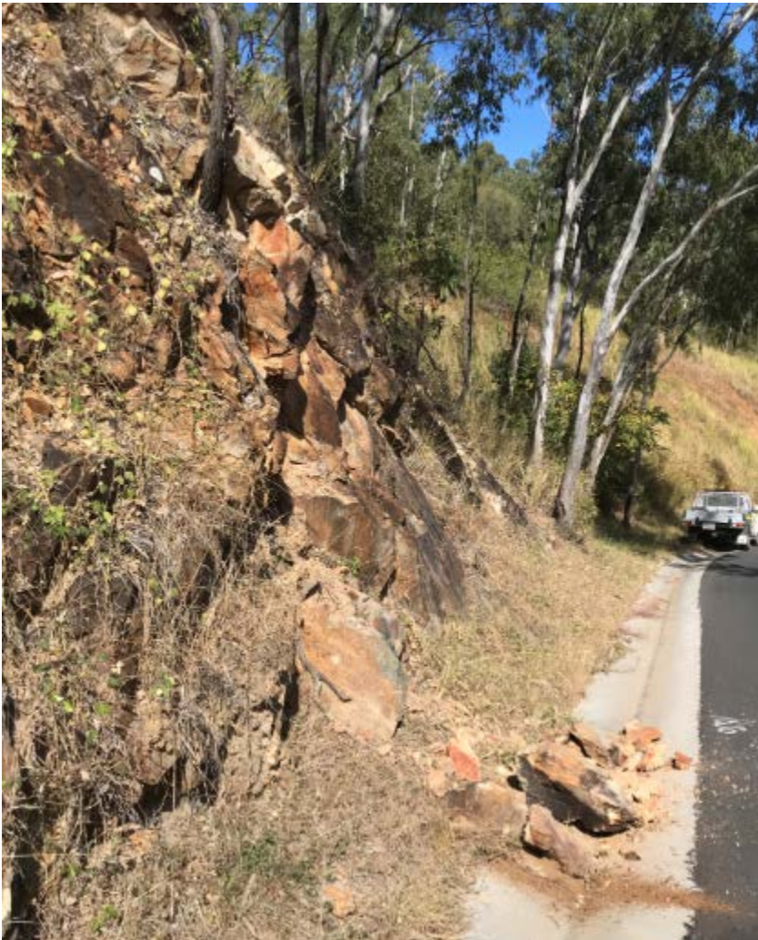
Figure 5-1 Small rock fall promoted by adverse dip and rootjacking by trees
