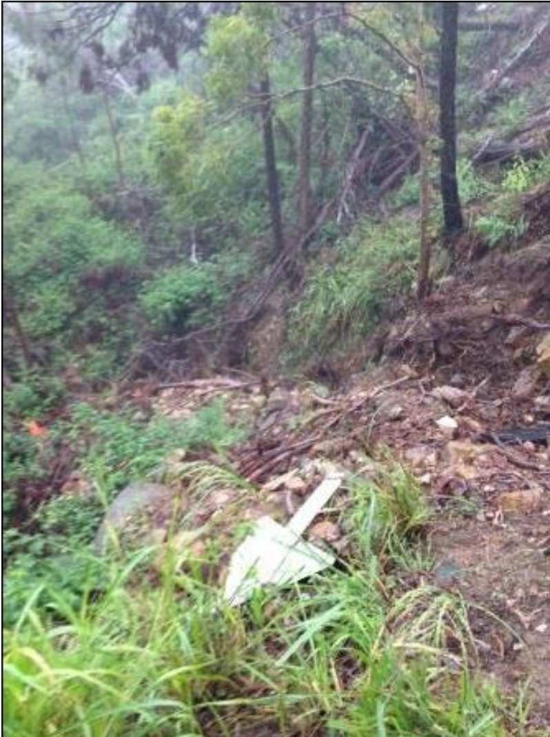
Figure 5-5 Small gully landslide; fluidised material caused by concentration of water flow
