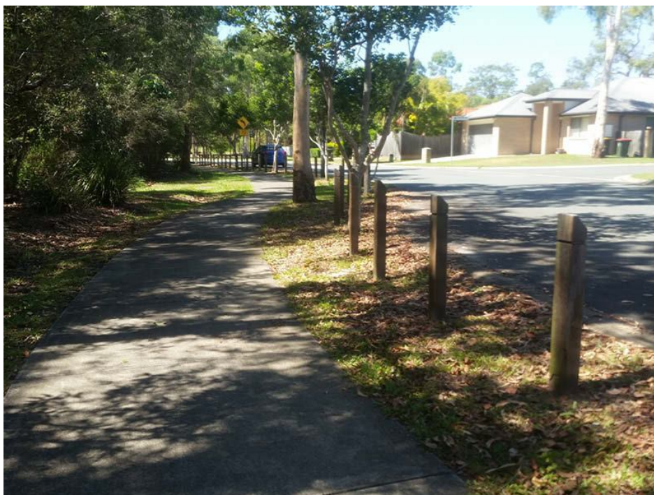
Figure 40: A buffer strip treating road runoff before it sheets over a footpath and into a swale
