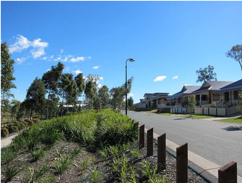
Figure 35: Example of a vegetated swale
