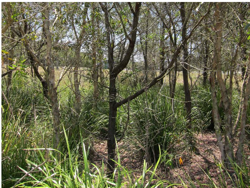
Figure 16: A bioretention system with turf on the batters shows no sign of weeds or grass in its centre
