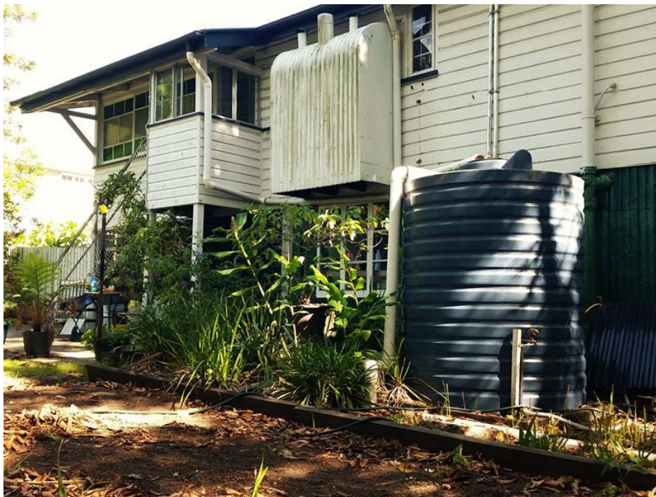
Figure 41: Example of a rainwater tank
