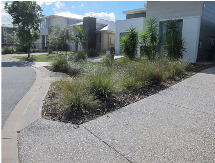
Figure 18: Low growing understorey plants in a streetscape bioretention system in the verge
