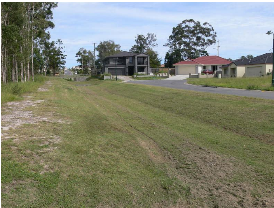
Figure 36: Example of a grass swale
