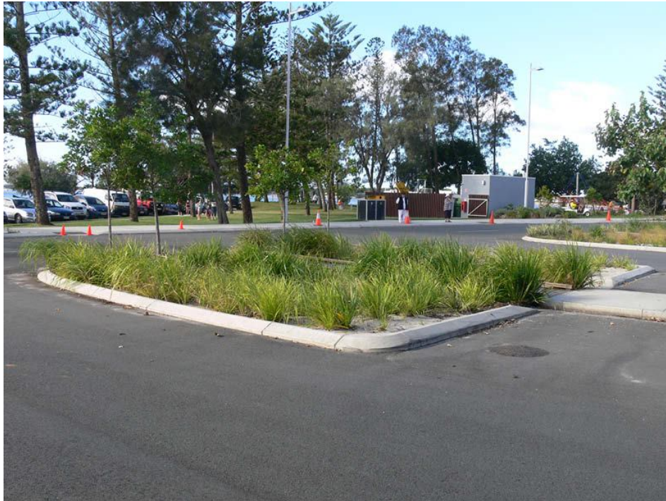
Figure 26: High profile streetscape bioretention system
