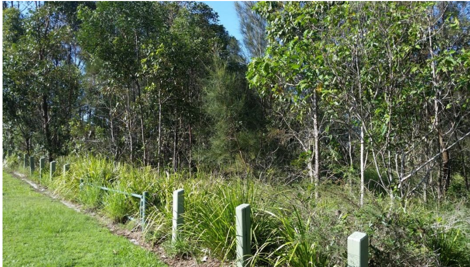
Figure 45: A bioretention system and a detention system co-located and planted to appear like a pocket of bushland
