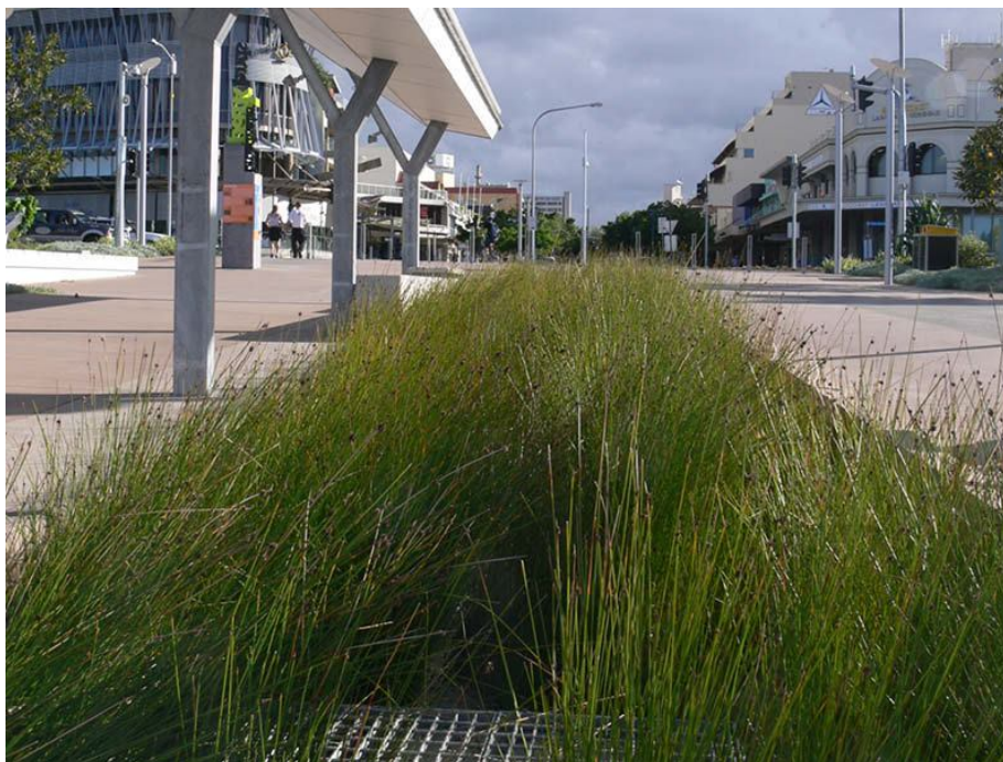
Figure 28: Bioretention system adjacent seating in a high profile parkland
