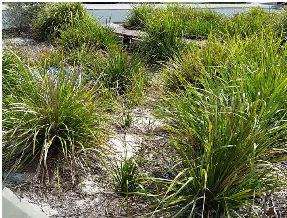
Figure 13: A bioretention system with bare space between Lomandras (bushland aesthetic not shown)
