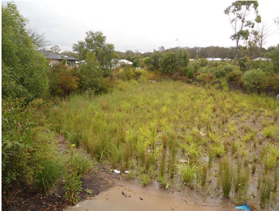
Figure 9: Precinct scale bioretention system co-located with a stormwater detention basin (bushland aesthetic not shown)
