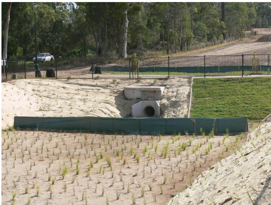
Figure 46: A combined bioretention and flood detention basin that is poorly integrated into the landscape and showcases a number of other aspects of inappropriate design.
