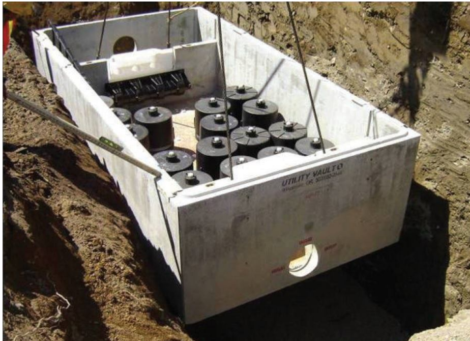
Figure 33: Example of a proprietary cartridge filter stormwater treatment system
