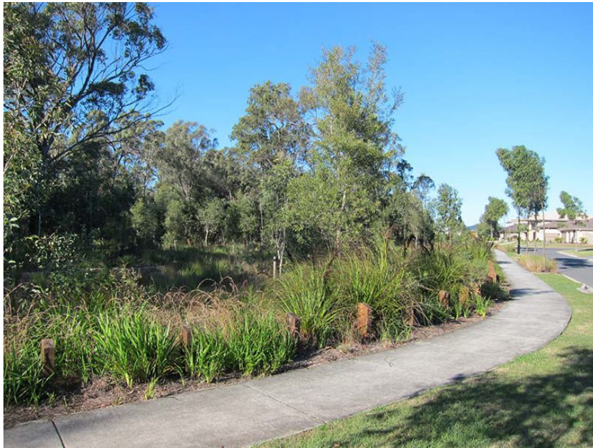
Figure 7: Precinct scale bioretention system adjacent to parkland
