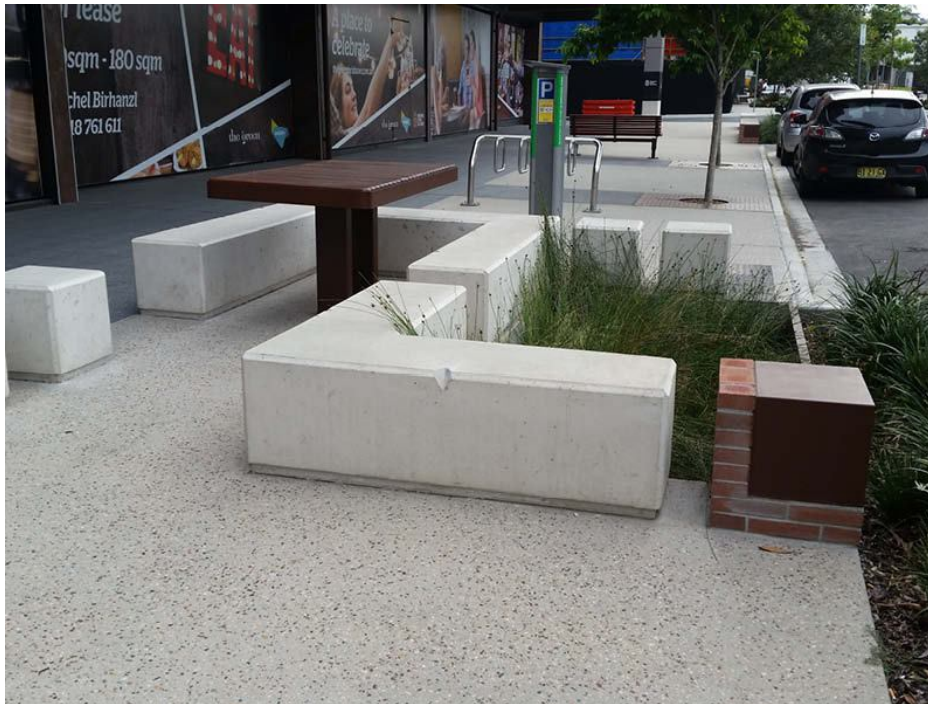
Figure 27: Bioretention system adjacent the road and seating in an inner city multi-storey residential development
