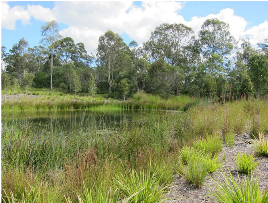
Figure 44: A sediment basin upstream of a bioretention system
