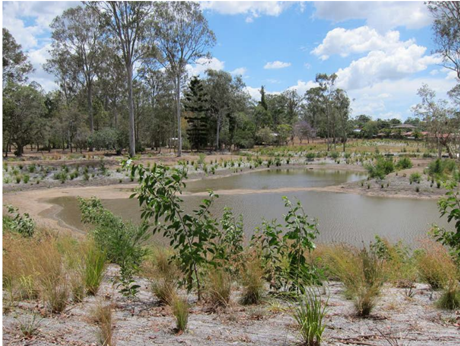
Figure 11: A very large flood detention basin showing newly planted pioneer and longer lived canopy species
