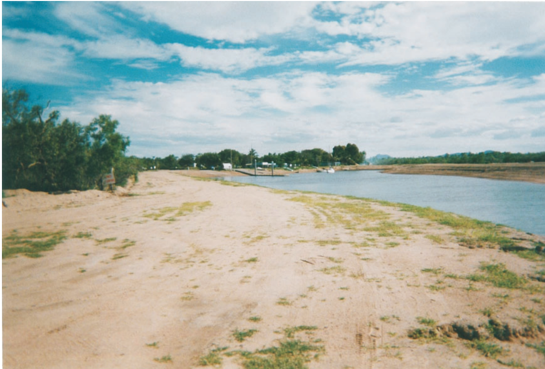
Molongle Creek Berth Facilities
