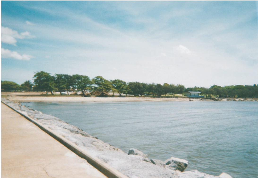
View to the North from Bowen Jetty to Bowen Foreshore
