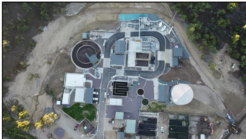
Bowen Sewage Treatment Plant
