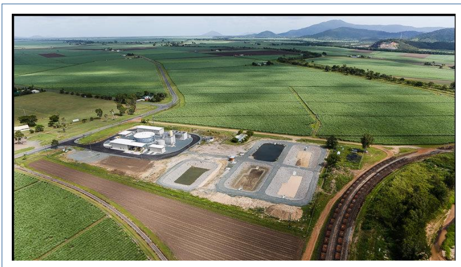
Proserpine Water Treatment Plant
