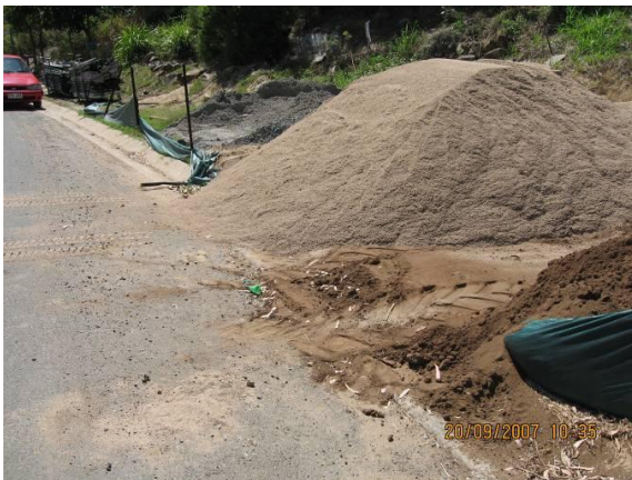
The stockpile must be located behind the sediment fence
