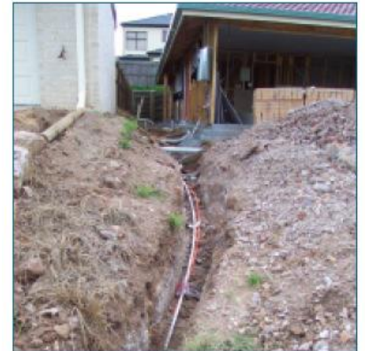
Service trenches should always be backfilled, capped with topsoil and compacted
