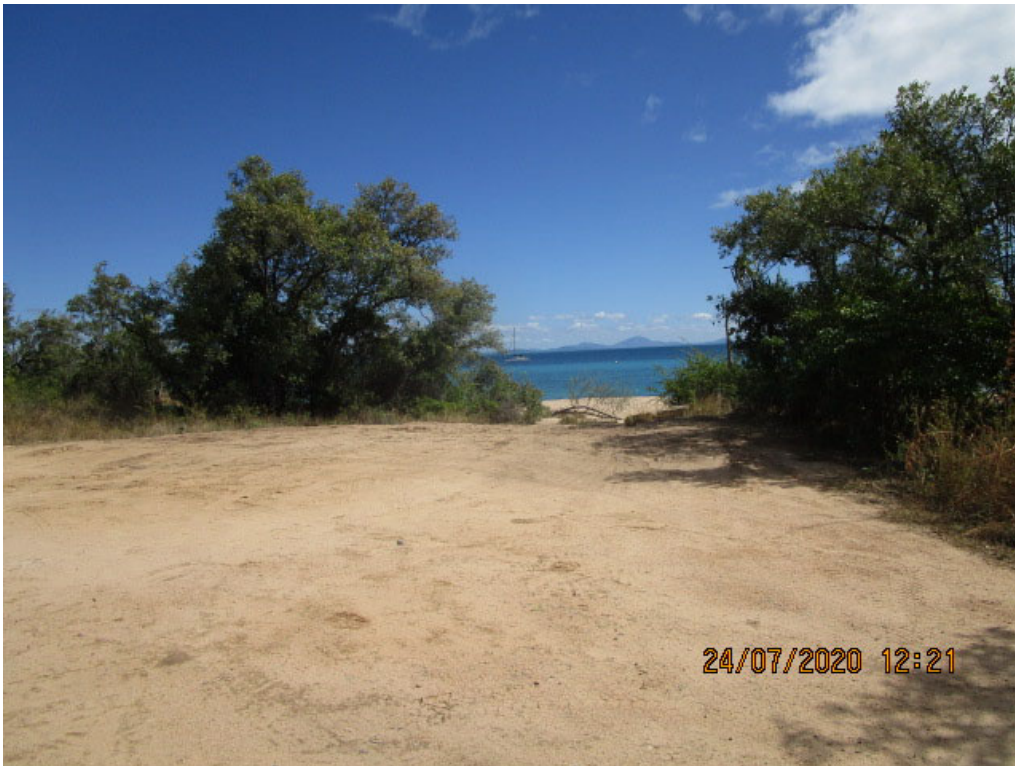
Figure 6: Area Cleared for Vehicle Parking and Beach Access
