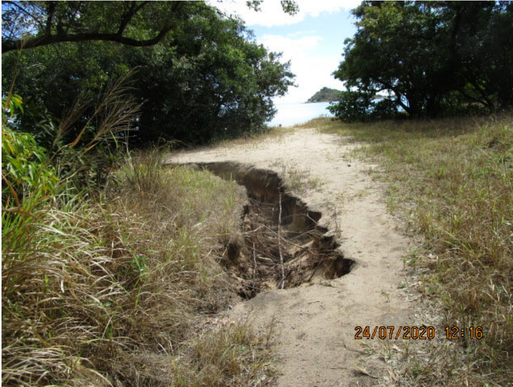
Figure 5: Erosion Caused by Vehicle Access to the Beach
